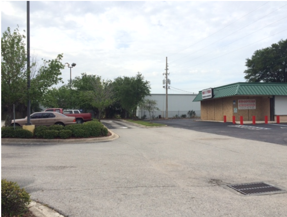
Proposed cross-connectivity access at Burger King parcel Source: Staff, Planning and Development Department Date: June 1, 2017
