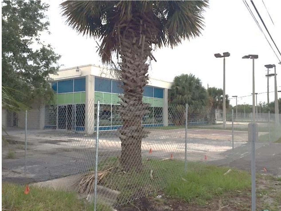
Subject Site – former automobile dealership, fronting Philips Highway Source: Staff, Planning and Development Department Date: June 1, 2017
